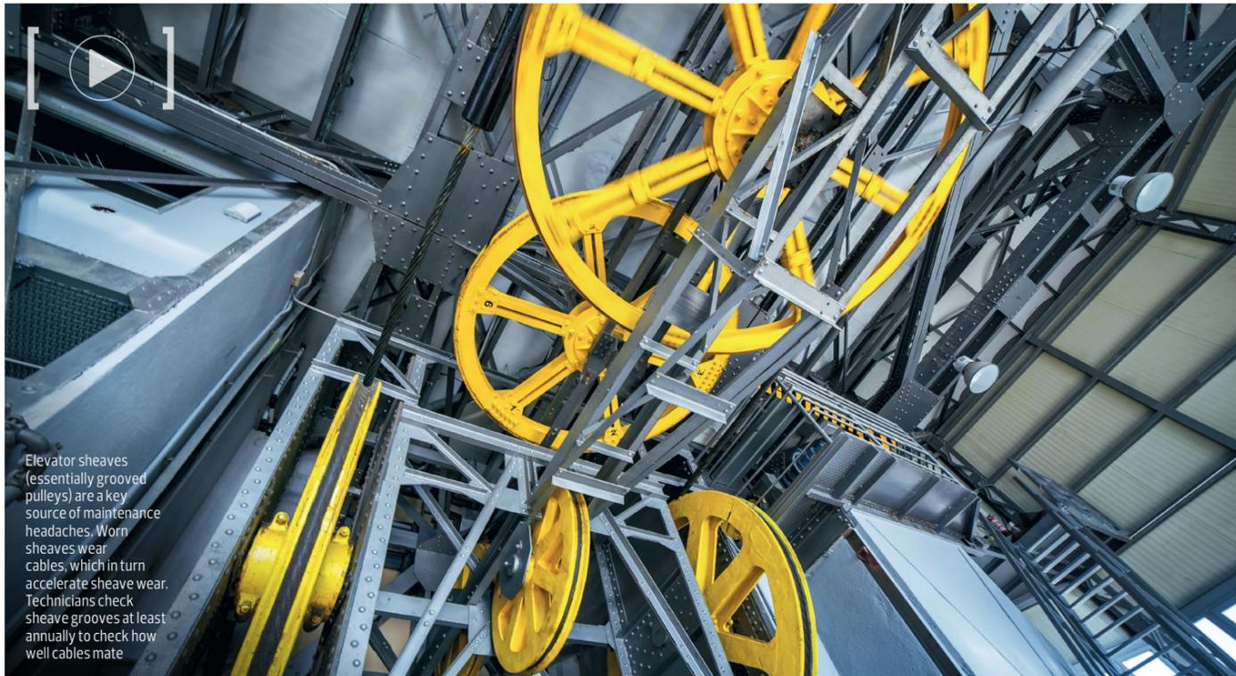
Elevator sheaves (essentially grooved pulleys) are a key source of maintenance headaches. Worn sheaves wear cables, which in turn accelerate sheave wear. Technicians check sheave grooves at least annually to check how well cables mate
